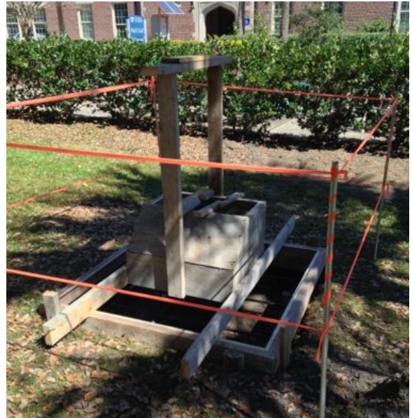
The base of the structure to hold the bent
